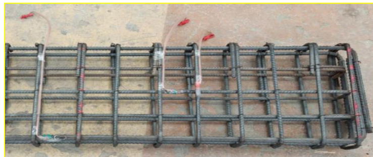
Fig. 3. Installation of strain gauges
