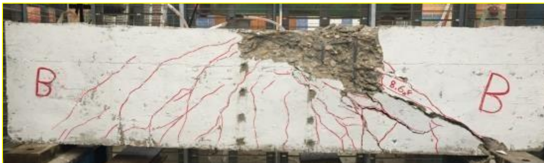
Fig. 5. Cracks pattern for experimental tested specimen B at failure
